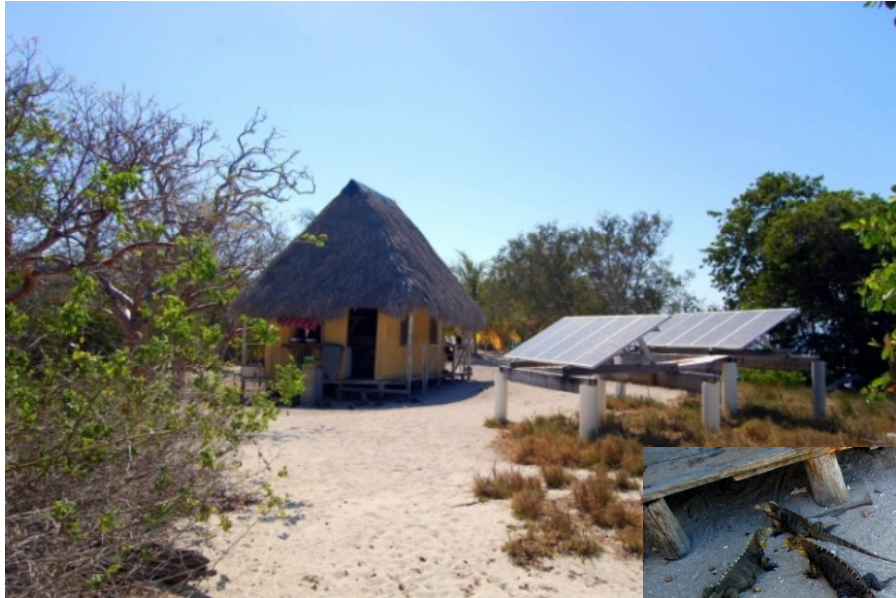
Beach restaurant at Cayo Machos (Note solar installation)
