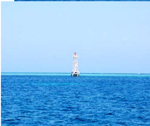
Lighted beacon at Cayo Restinga
