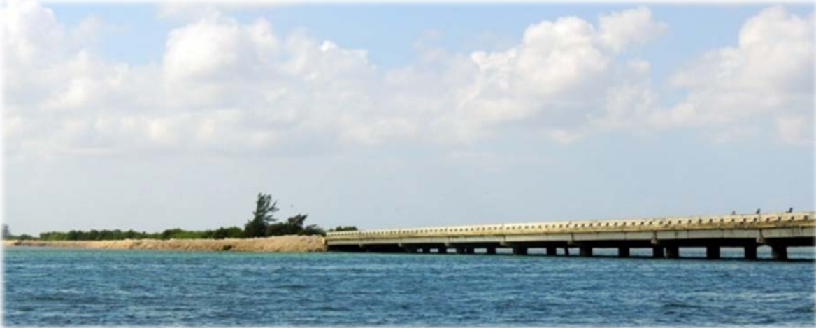
One of the 14 bridges along the “pedraplén”
