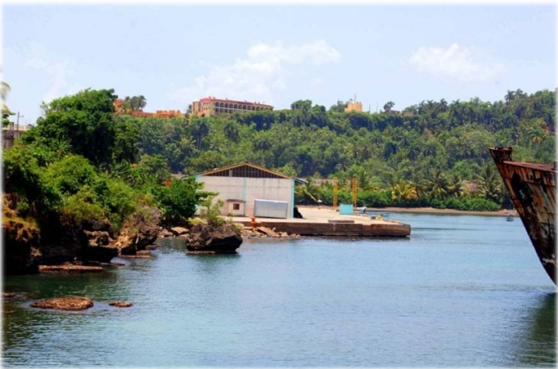
Commercial dock and Guardafronteras post; wreck to right and Hotel Castillo on top of hill
