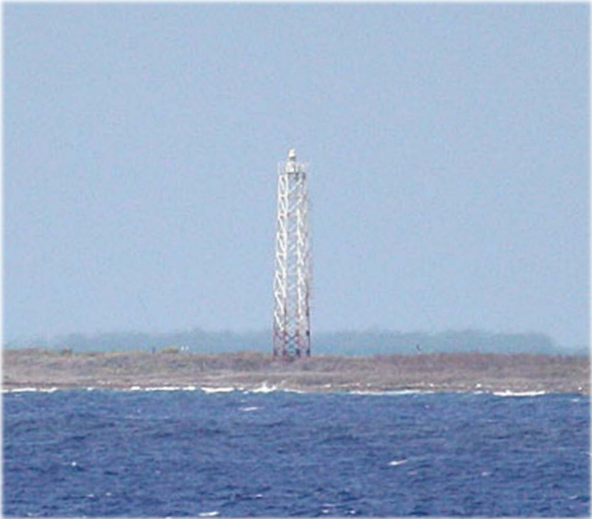
Cayo Confites is marked by a white lattice tower, 66' tall, that flashes white every 7.5 seconds
