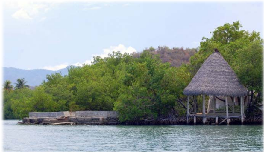
Concrete jetty by the hatched roof palafito
